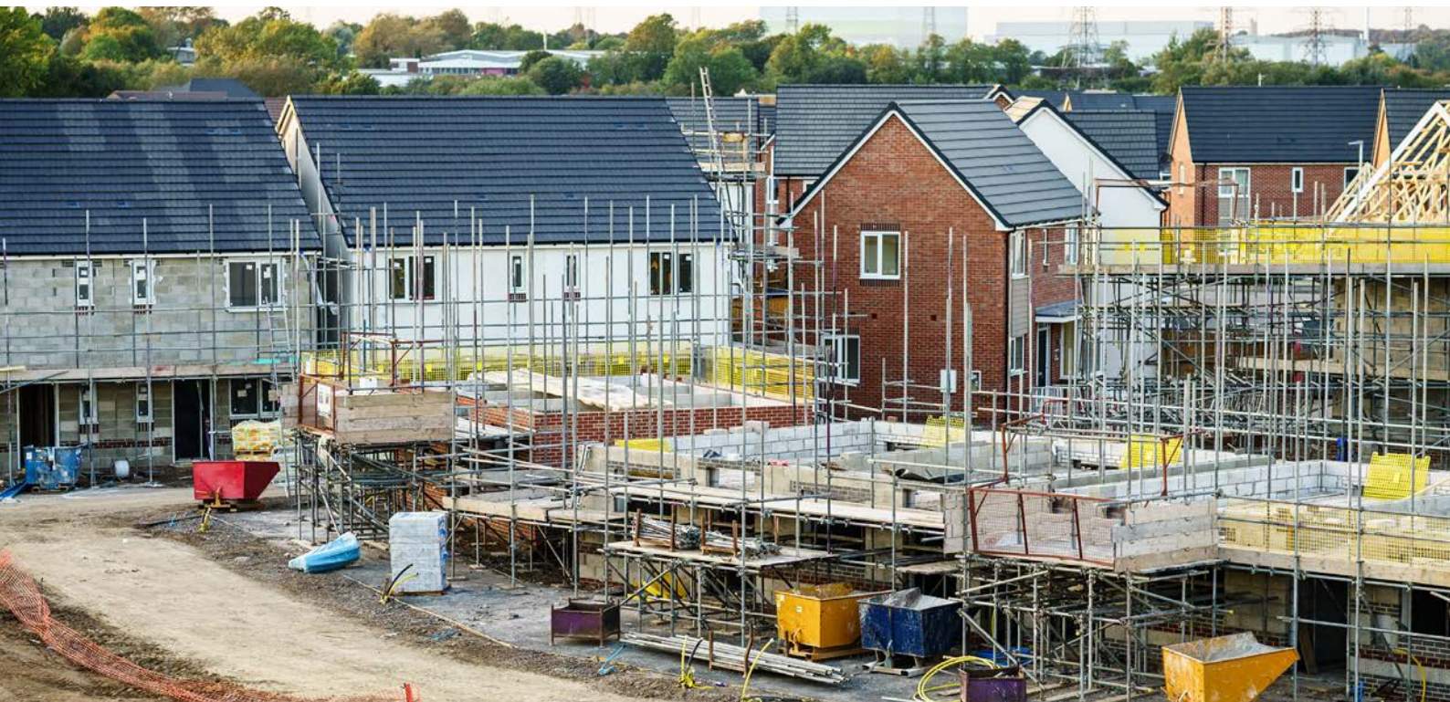
OAHF homes under construction in Pinhoe, Devon
