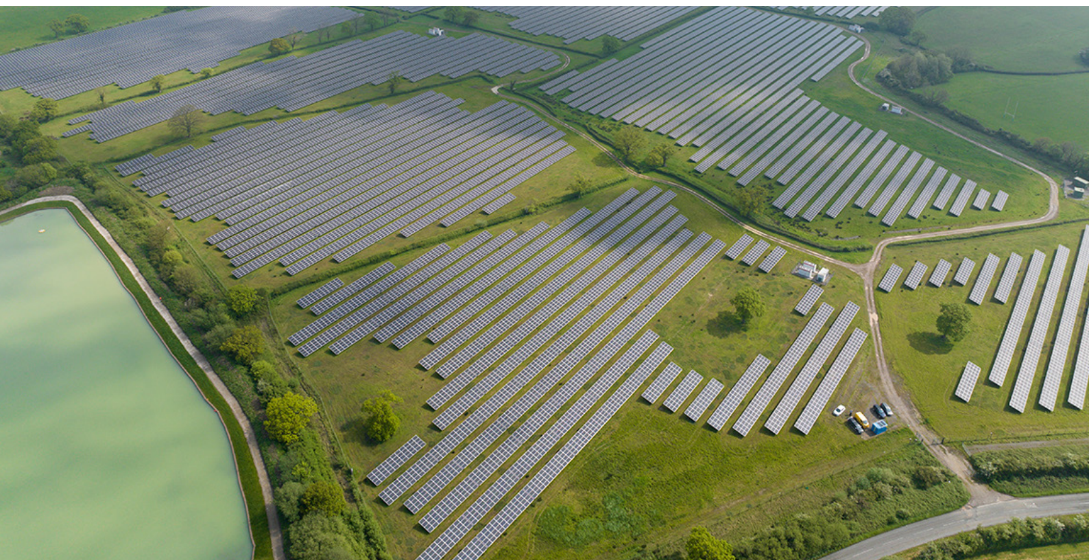
Wessex Gardens solar farm, Grange Farm, South Gloucestershire
