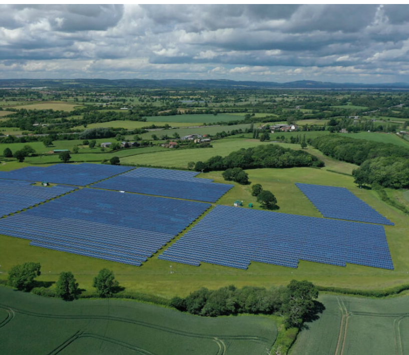
Wessex Gardens solar farm in Upper Wick, Stroud
