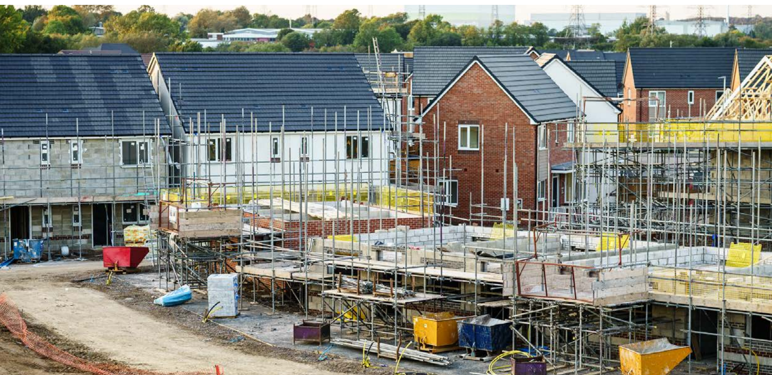
OAHF homes under construction in Pinhoe, Devon
